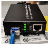
Wan port operational
